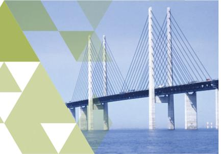
Most of the bridge parts were made on the mainland and then floated out to the construction site for assembly.
