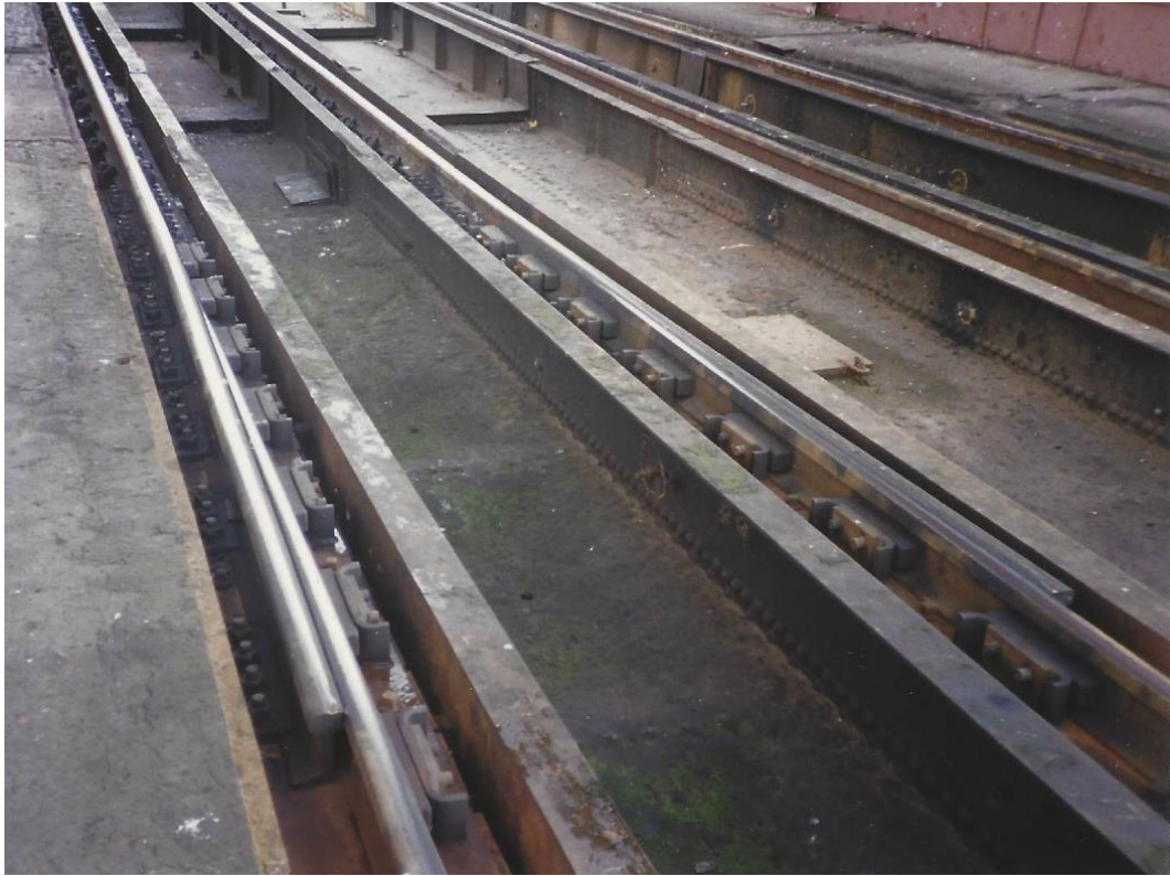
Figure 14.1 'Forth Bridge' expansion switches. At FB on Figure 14.3
