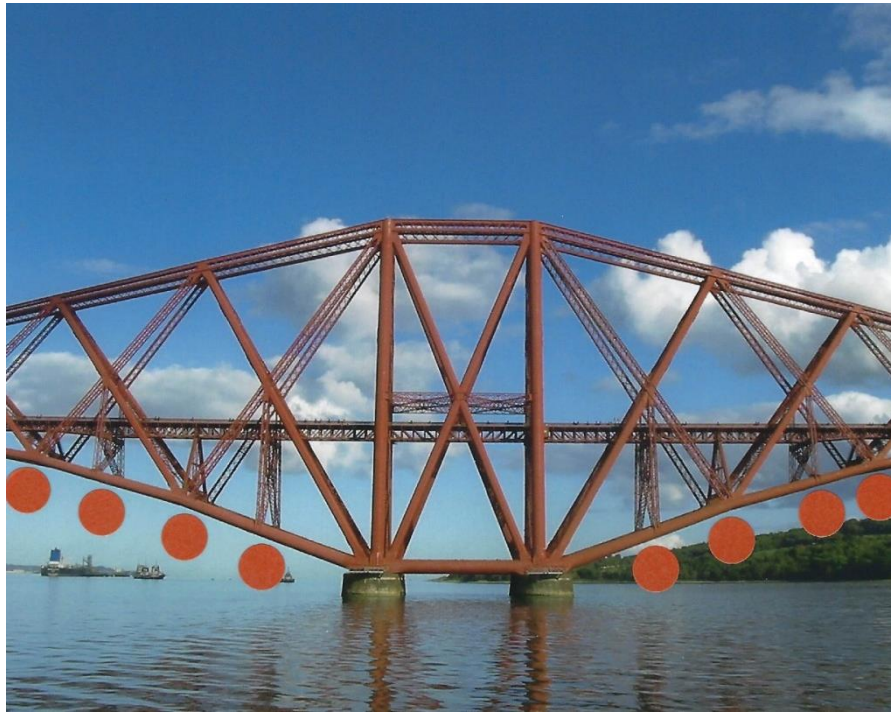
Figure 6.7 The Internal Railway Viaduct is supported by trestles resting on the bottom booms (struts) at the locations shown by a circle.
