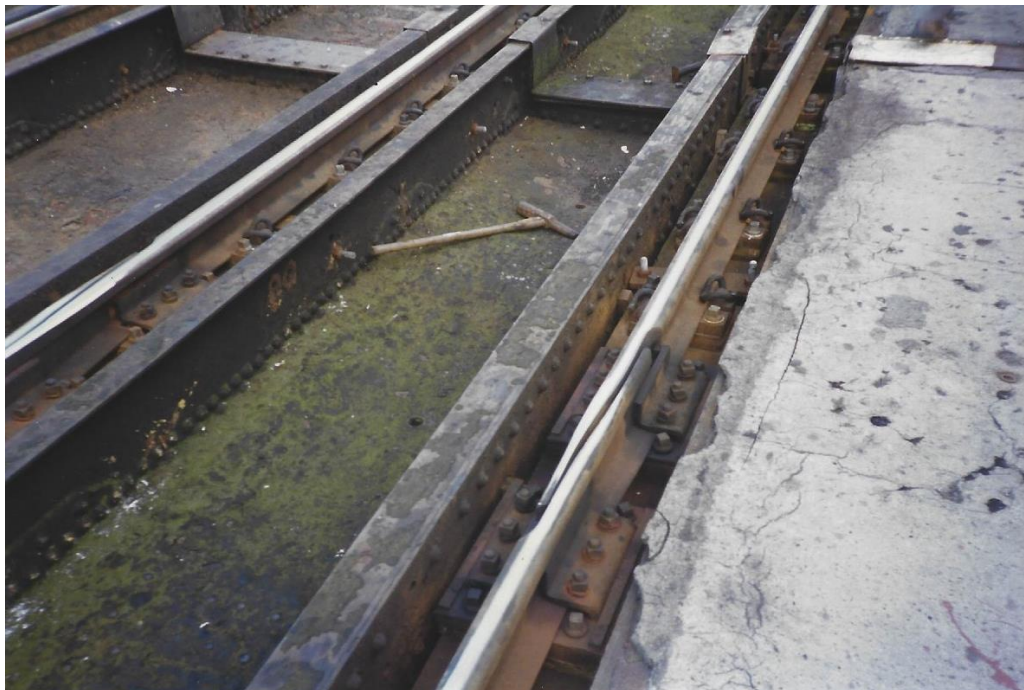
Figure 14.2 Standard expansion switches. At S on Figure 14.3.
