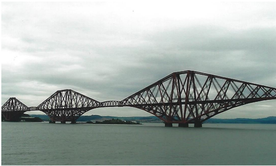
Figure 6.2 the Cantilevers including two Central Girders (the Cantilever Section) (It is the Cantilever Section that makes the Forth Bridge such an unusual and interesting structure).
