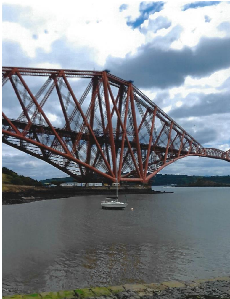
Figure 17.4A Cross bracing between Compression members (struts) is clear in this view from North Queensferry of the Fife Cantilevers.
