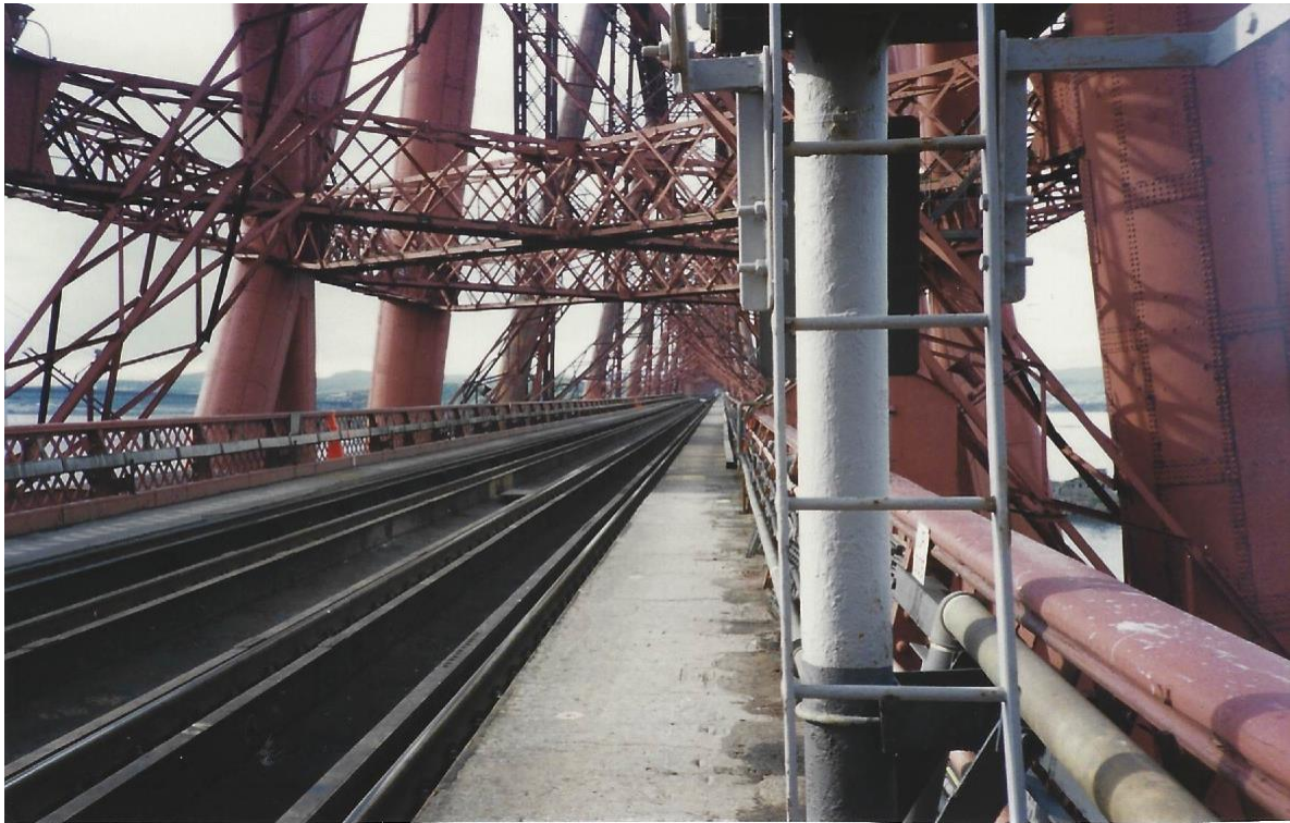
Figure 6.5 The internal railway viaduct has two tracks and walkways for maintenance staff. The paint used on the Forth Bridge has always been red in colour.
