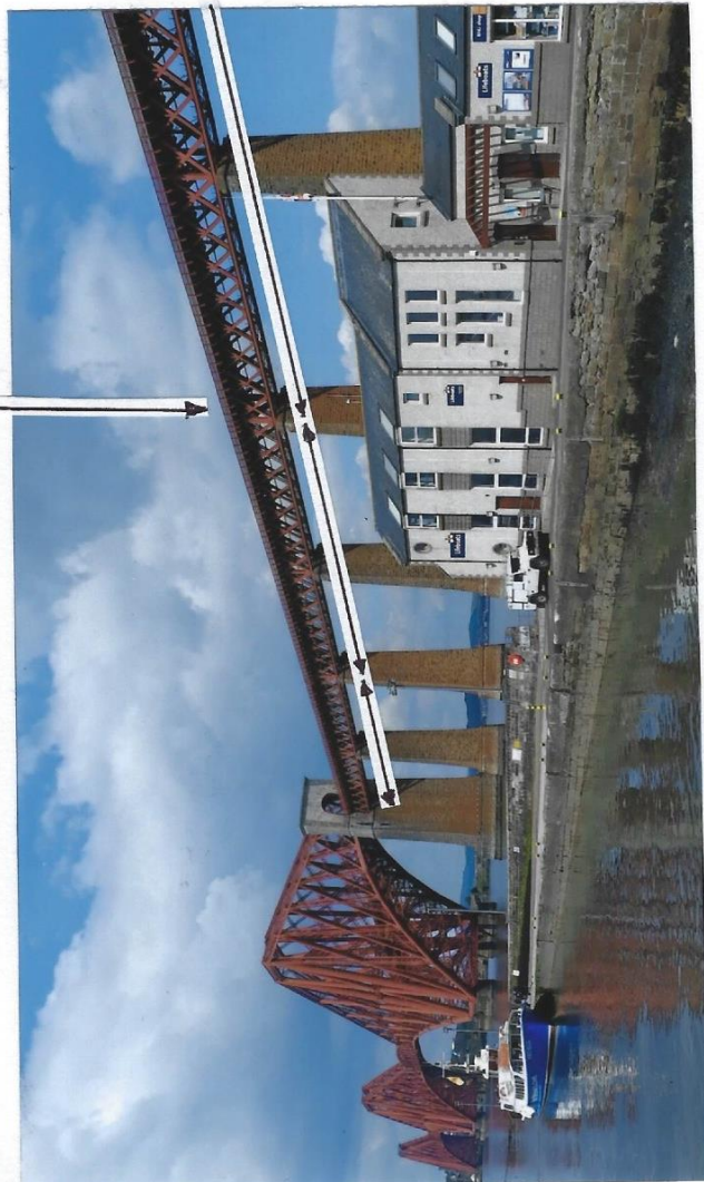
Figure 19.4 The arrows indicate the continuous spans - Queensferry Approach Viaduct
