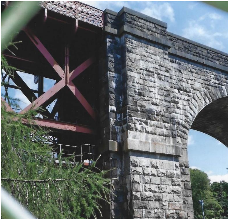
Figure 19.5 The connection between the Queensferry Approach Viaduct and the adjoining masonry arches. Several multi-span steel bridges have their extreme ends bearing on masonry or brick arches located on firm ground. The south end of the Tay Bridge at Wormit is another good example. (See also Figure 5.2)
