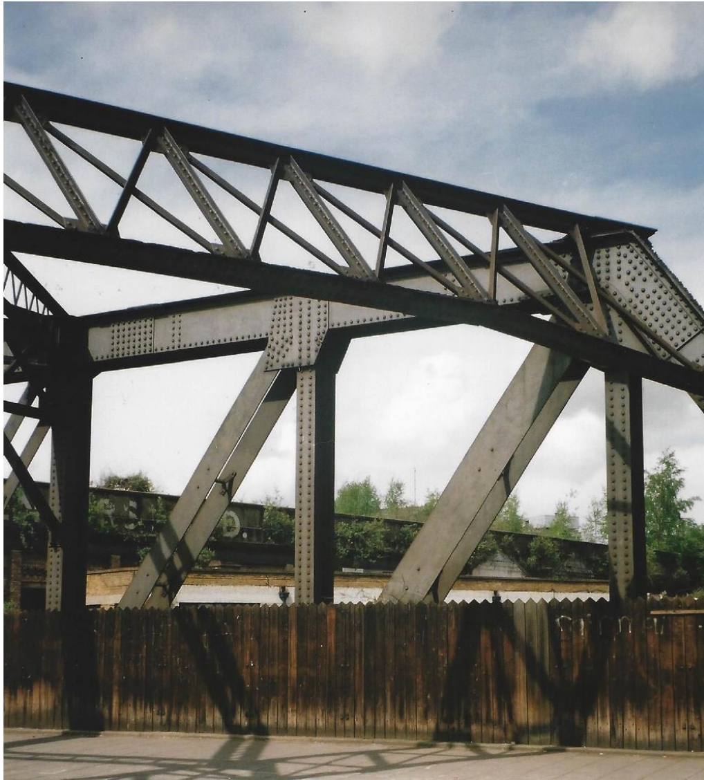
Figure 18.2 A bridge with members connected by many rivets
